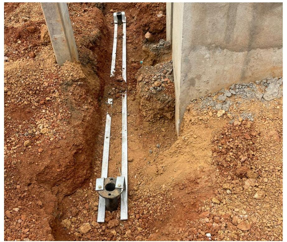
PLACING AND FIXING OF PANEL BOARDS ALONG WITH EARTHING IS PROGRESS
