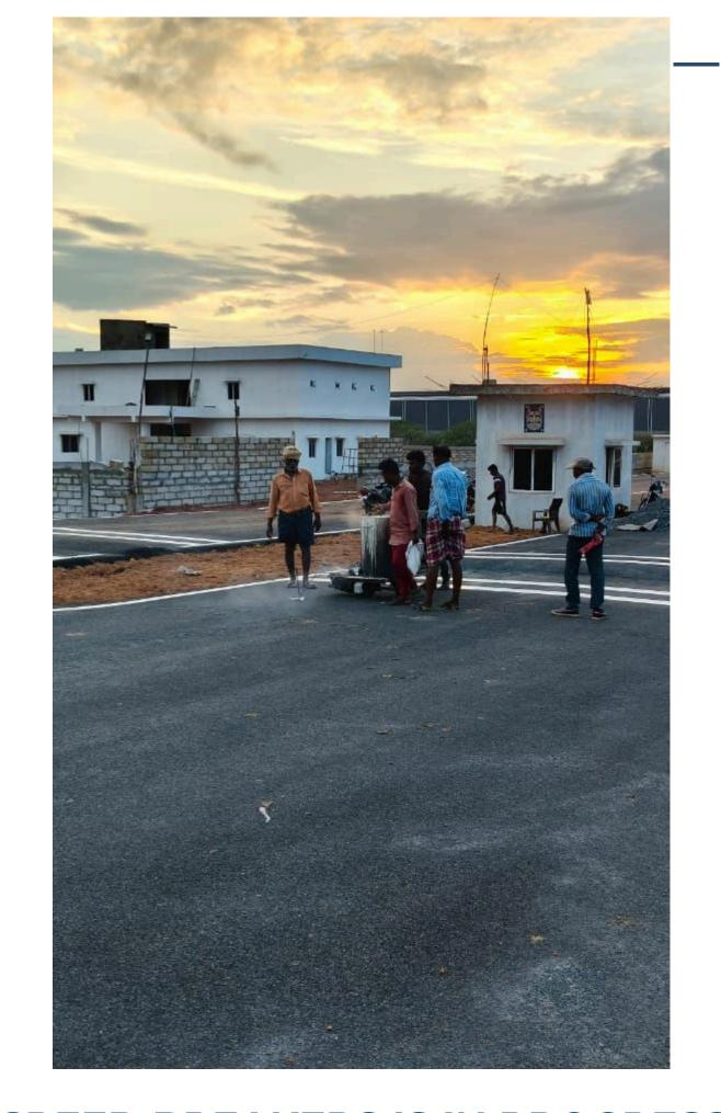
MARKING OF WHITE LINES ON BT ROAD AND PAINTING OF SPEED BREAKERS IS IN PROGRESS
